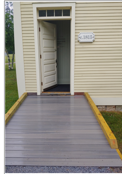
The newly constructed accessible ramp at the Log Schoolhouse entryway. (Photo by Bonnie Potter)
