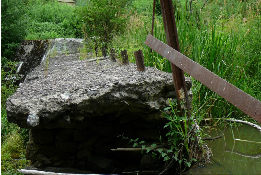
Figure 23. View east of the concrete cap on the secondary spillway section (stone masonry portion) of the Mill Pond Dam.
