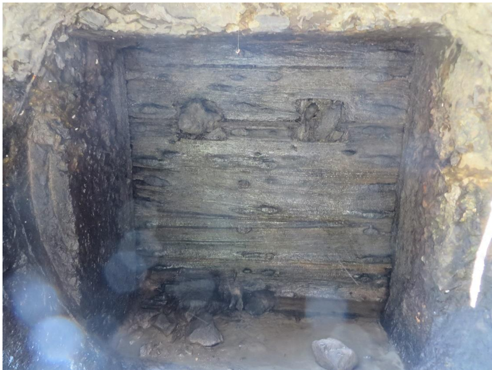
Figure 30. View southeast of wooden boards within the low outlet gate opening in the primary spillway section of the Mill Pond Dam during deconstruction.
