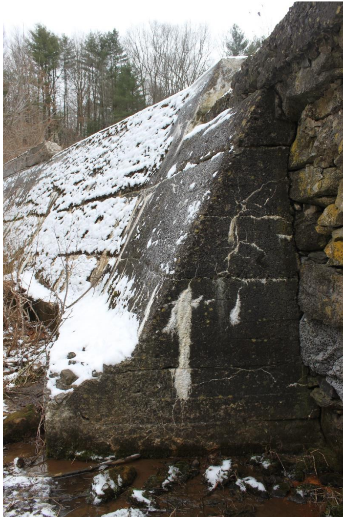
Figure 37. View east of the concrete “buttress” at the junction between the stone masonry and the mass concrete sections of the Mill Pond Dam.
