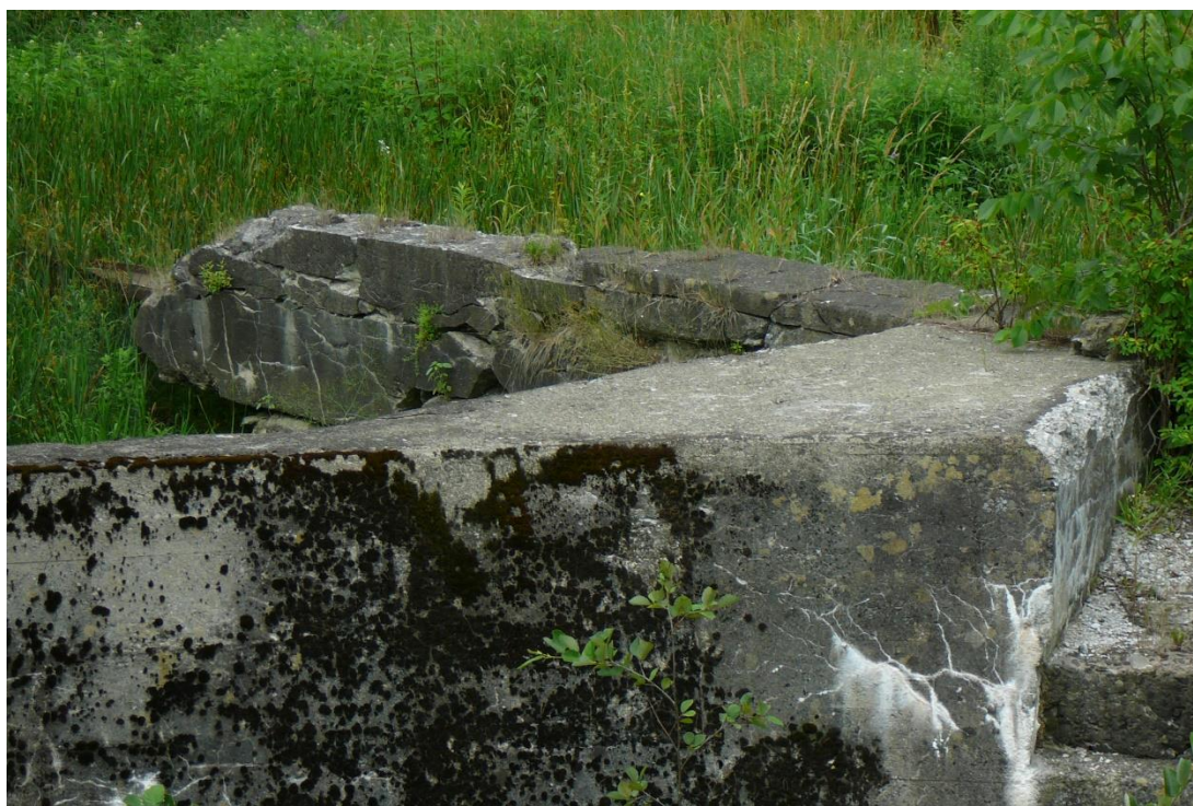
Figure 41. View south of west portion of possible training wall looking over the top of the mass concrete section of the right (east) wing of the Mill Pond Dam.
