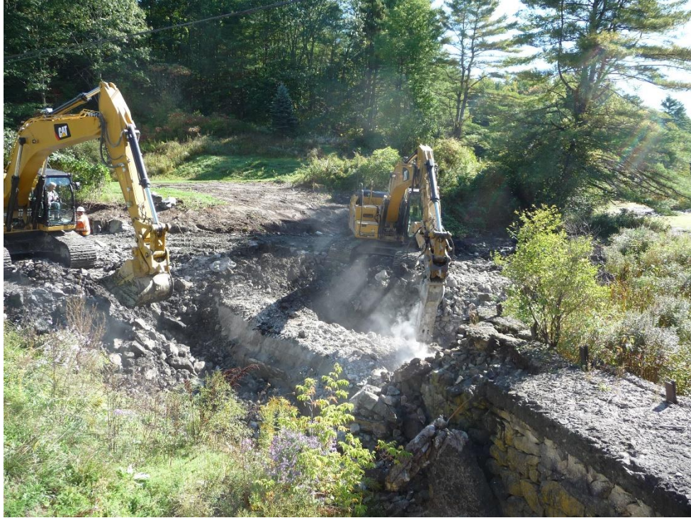
Figure 38. View southeast during the deconstruction of the mass concrete section of the right (east) wing of the Mill Pond Dam.
