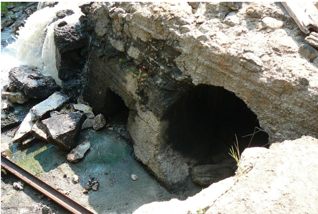
Figure 28. View east of the primary spillway section of the Mill Pond Dam during deconstruction with low outlet gate (left) and penstock (right) openings exposed.
