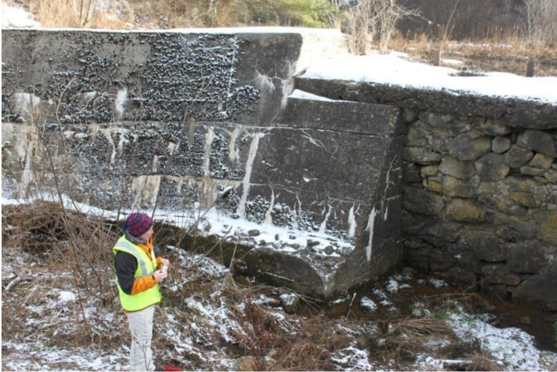
Figure 34. View east of the junction between the stone masonry and the mass concrete sections of the Mill Pond Dam; note concrete “buttress” at center.
