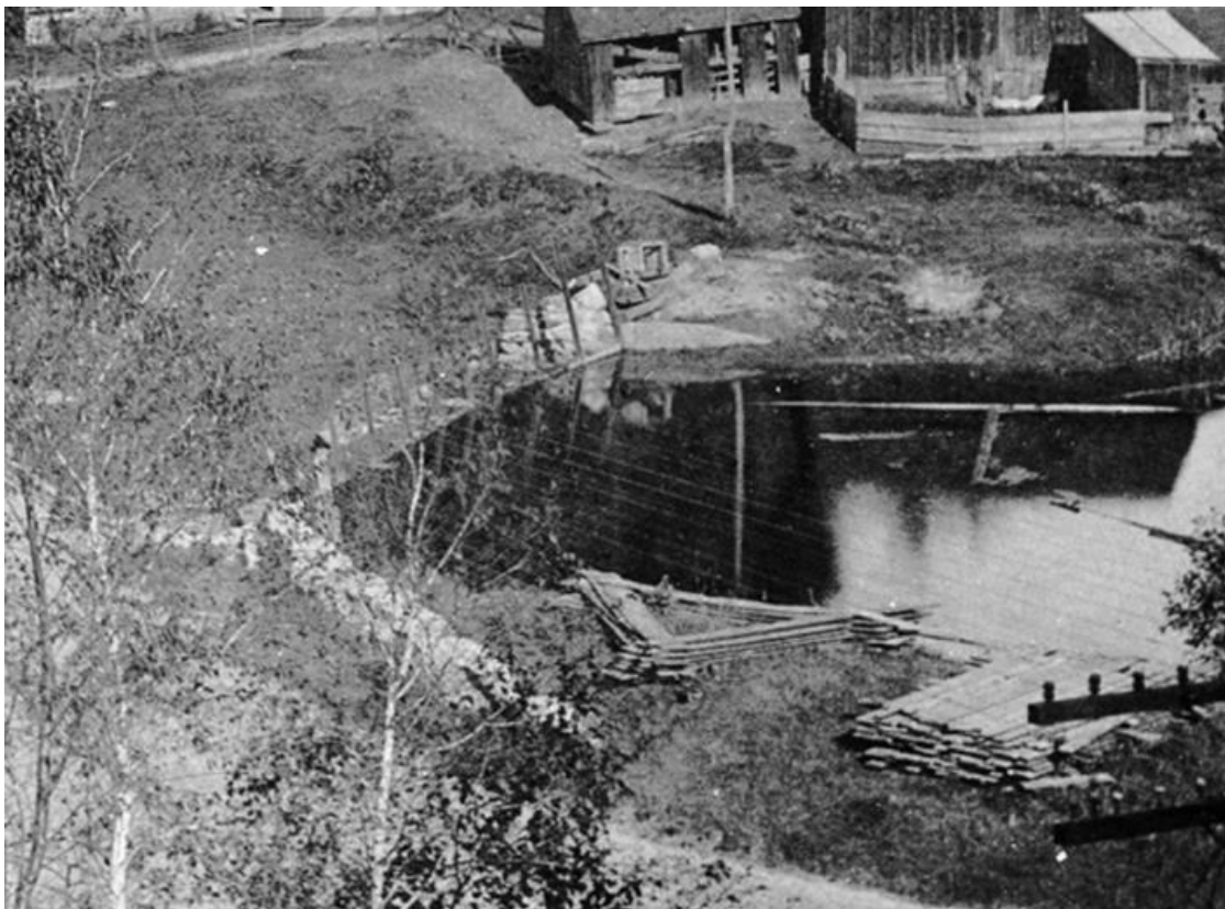
Figure 26. Detail of historic photographic postcard (see Figure 14); note railroad rails in place and stone structures at the left (west) and right (east) wing, and abutment areas.
