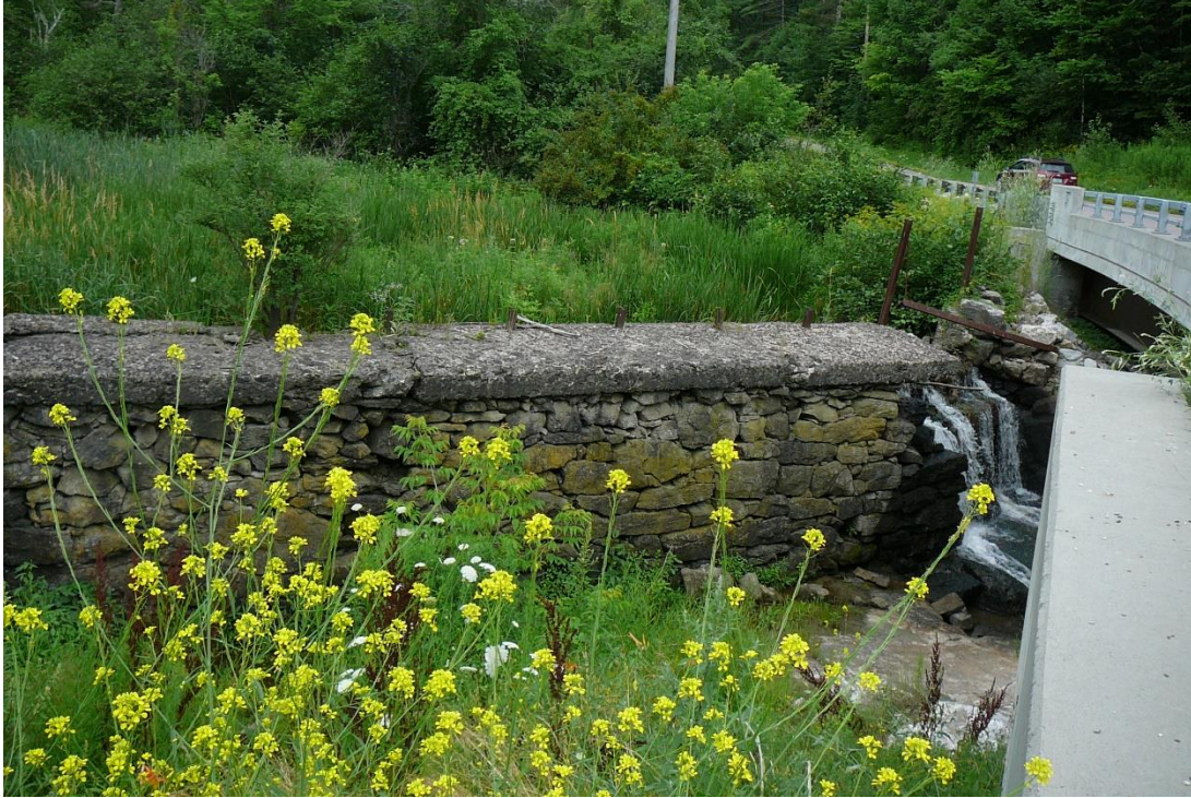
Figure 21. View southwest of the secondary (stone masonry portion) and primary spillway (breached portion) sections of the Mill Pond Dam.
