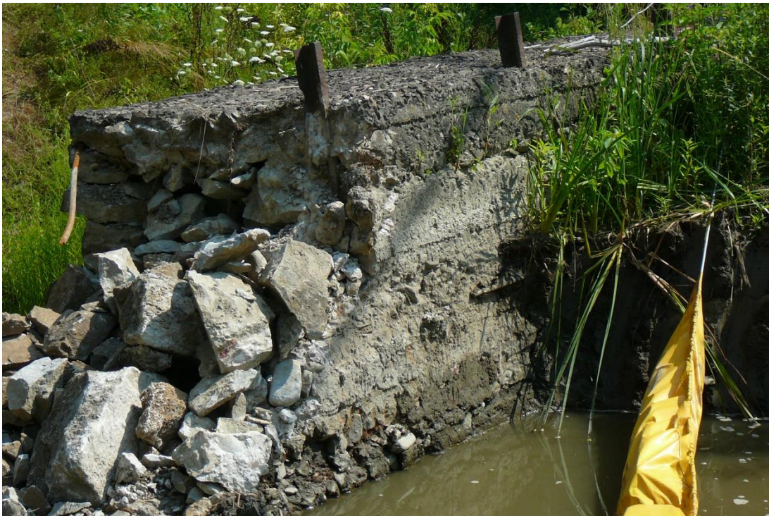
Figure 24. View east of the concrete cap and upstream facing on the secondary spillway section (stone masonry portion) of the Mill Pond Dam, during deconstruction.
