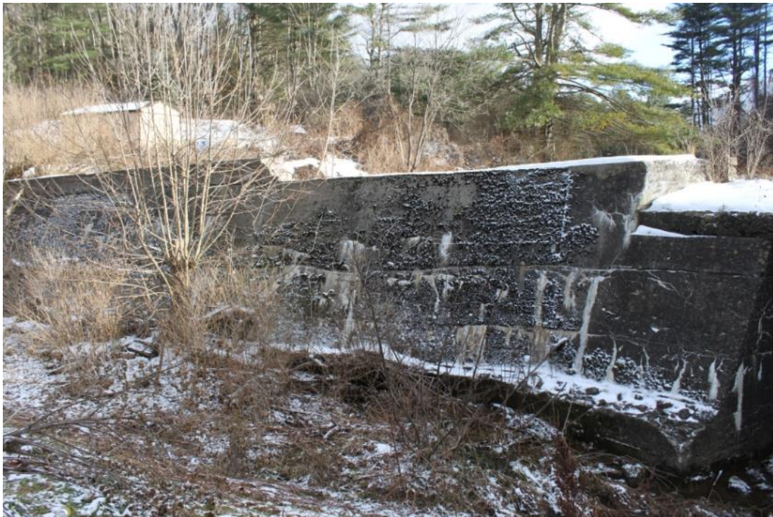
Figure 33. View east of the mass concrete section of the right (east) wing of the Mill Pond Dam.
