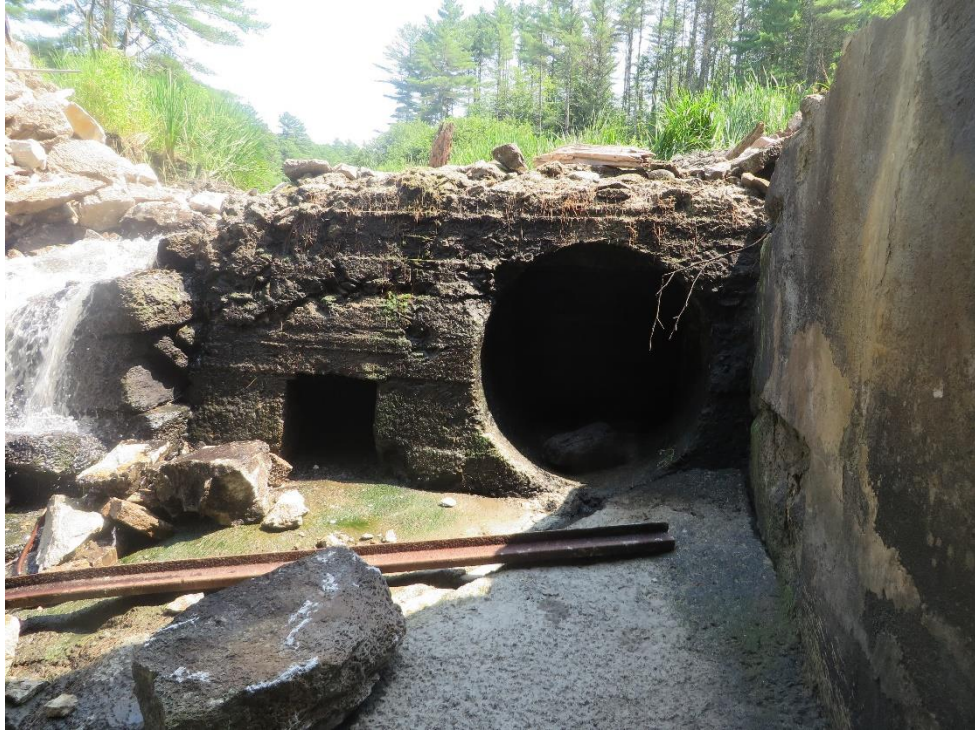
Figure 29. View southeast of the primary spillway section of the Mill Pond Dam during deconstruction with low outlet gate (left) and penstock (right) openings exposed.
