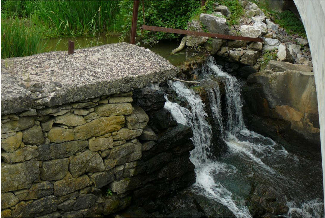
Figure 27. View southwest of the breached primary spillway section of the Mill Pond Dam, from Bridge No. 12.
