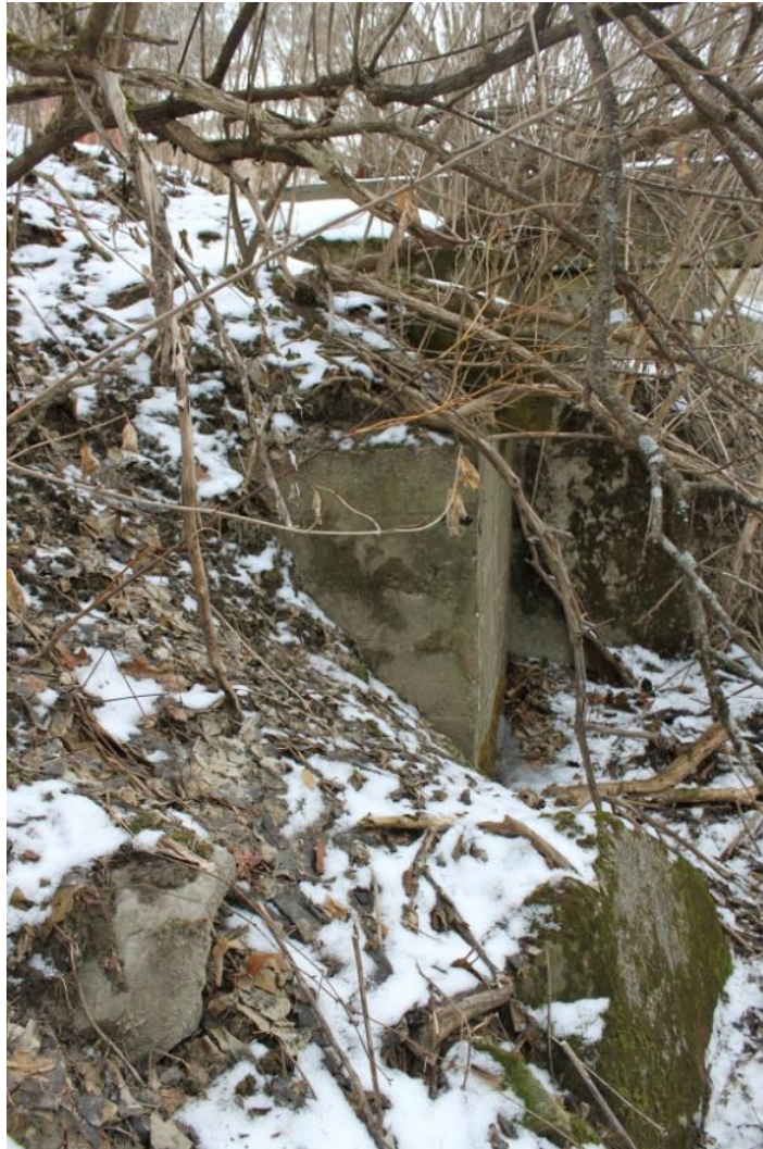
Figure 36. View southeast of the downstream side of the right (east) wing and abutment area of the Mill Pond Dam showing the concrete stepped baulk partially buried in the bank.
