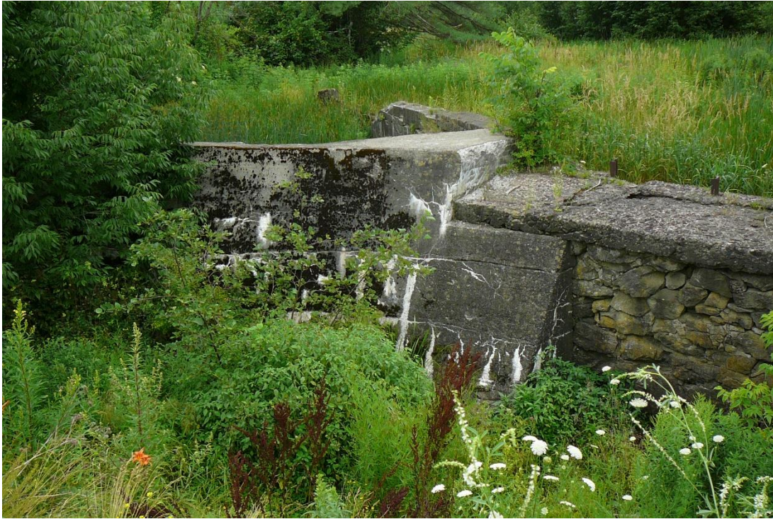
Figure 32. View southeast of the Y-shaped right (east) wing of the Mill Pond Dam; secondary spillway section (stone masonry portion) at right.
