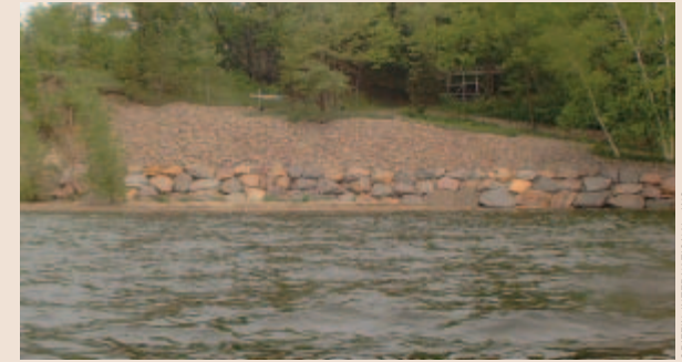
A stone riprap revetment combines smaller placed rocks on the face of the bank and larger rocks to help stabilize the toe of the bank near the waterline.
