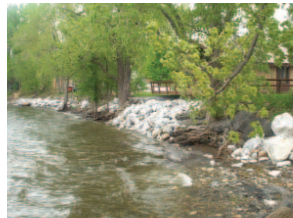
Construction of an erosion stabilization project may result in a stretch of shoreline becoming covered with unsightly stone riprap and causing erosion elsewhere.
