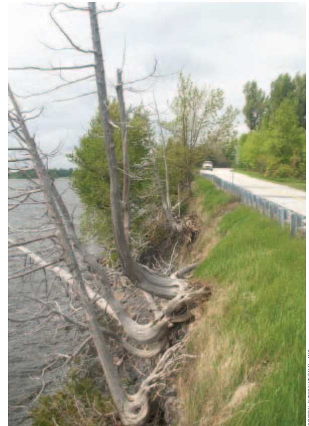
Paved roadways built along the shores of a lake increase the velocity of stormwater runoff that accelerates bank erosion.
