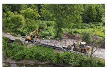
the road as needed to ensure thru traffic was accommodated as much as possible. The temporary bridge was delivered to the site in parts and sections, and the DPW Highway Crew worked together to assemble the bridge and move it into place. The project was completed according to plan and within the expected timeframe, thanks in very large part to the excellent teamwork exhibited by the DPW Highway Crew.
