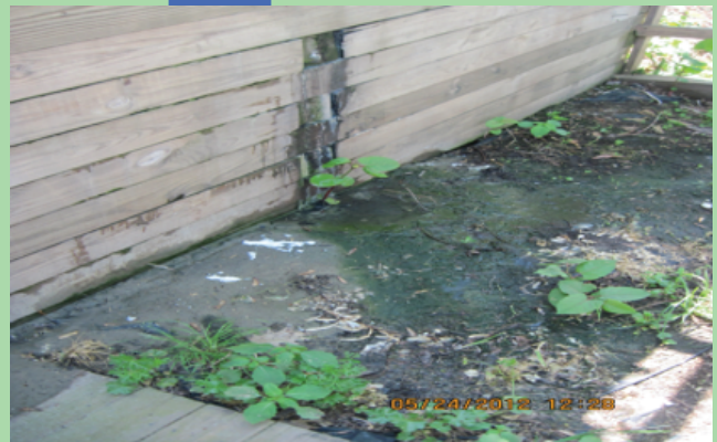
Failed “best fit” replacement septic system in Malletts Bay less than one year after installation.
